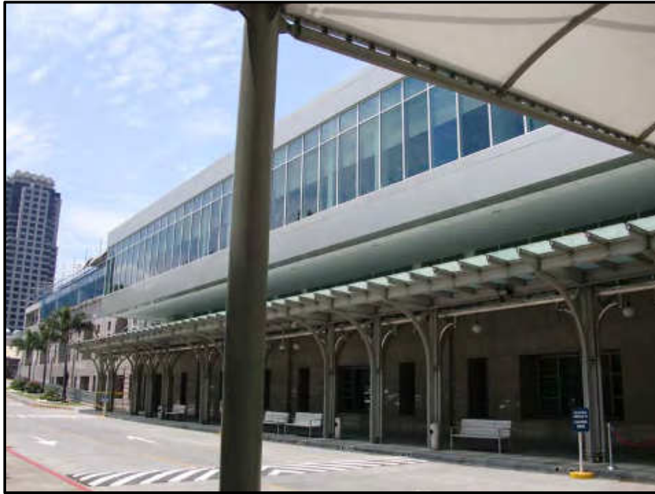
Photograph A7.5: Mezzanine Exterior (May 2010)
