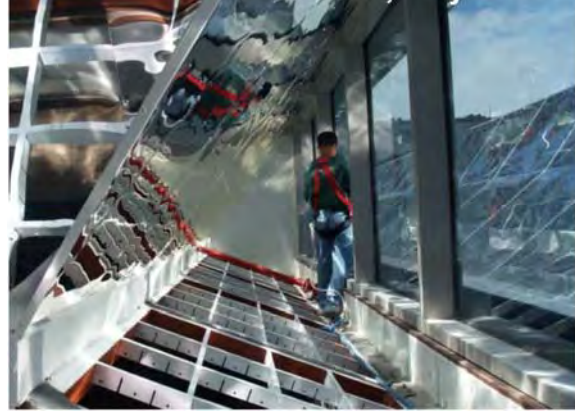
Photograph A8.6: Clerestory Cavity
