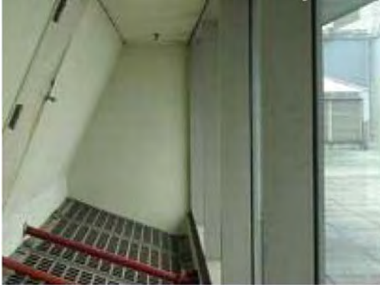
Photograph A8.5: Clerestory Cavity
