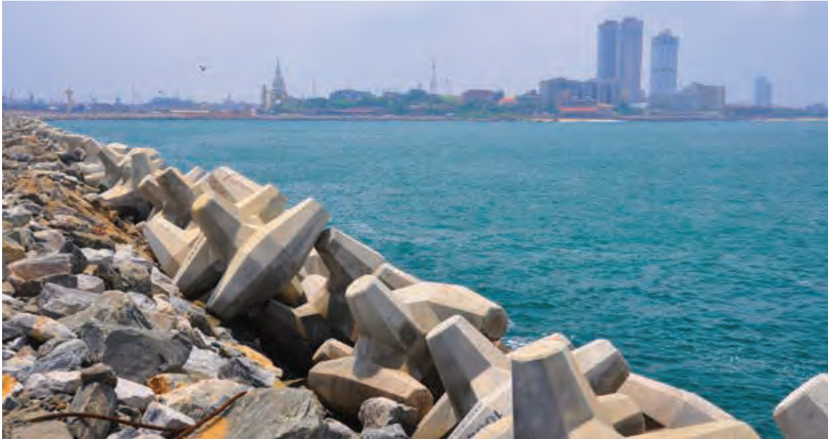
34,500 core-locs were used for the 6.4 kilometer-long breakwater. James Hutchison | ADB Photo Library.
