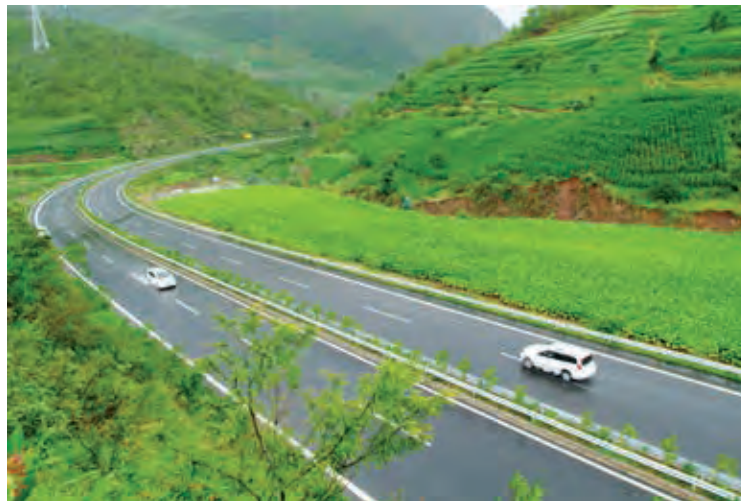
The project built a four-lane expressway that helped connect the remote province of Western Yunnan to markets and basic services.
