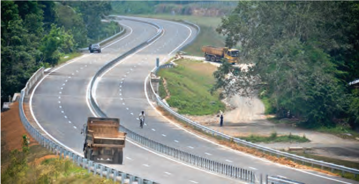
The ADB-financed section of Sri-Lanka's first limited-access expressway, the Southern Transport Development Project. James Hutchison | ADB Photo Library.
