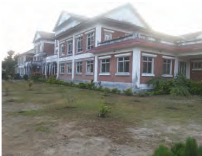
Kakarbhitta Inland Clearance Depot Passenger Terminal Administration building. ADB Photo Library.
