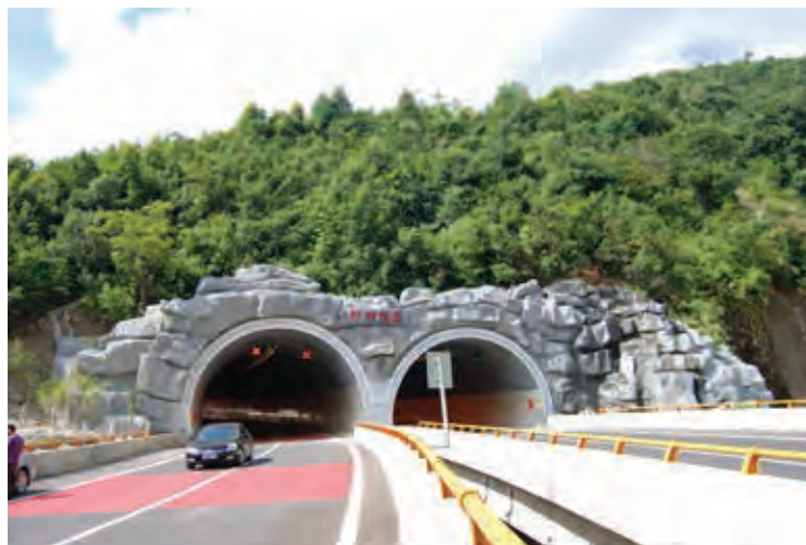
The tunnels of the expressway pass through mountains, while the bridges span deep valleys, rivers, and tributaries below.
