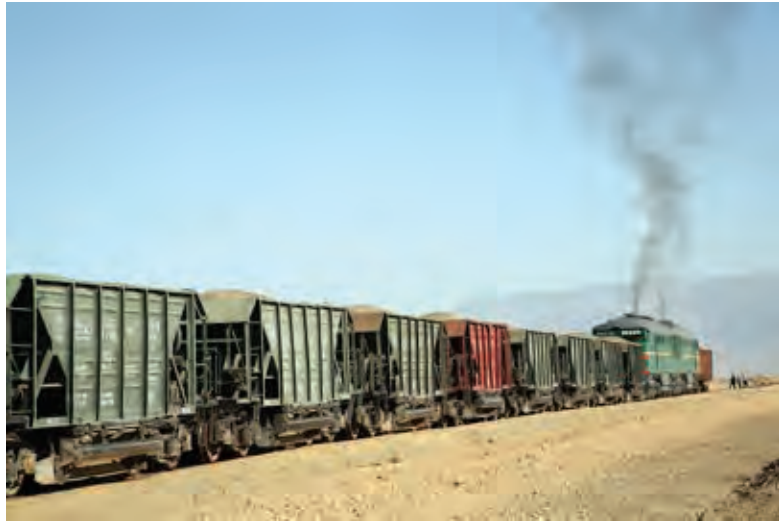
The 75-kilometers railway connects Mazar-e-Sharif town to the trade gateway of Hairatan and to the rest of Afghanistan. Ash Sweeting | ADB Photo Library.
