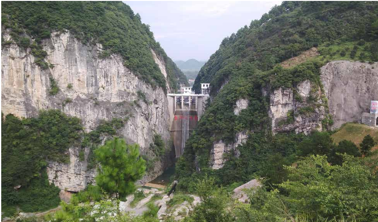
Yudongxia Dam and Reservoir.
