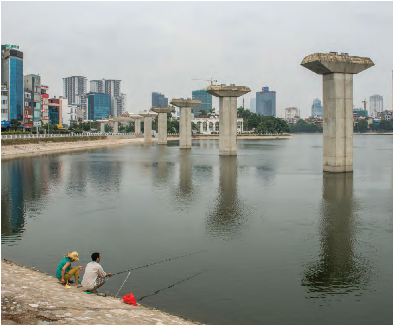
Ha Noi Metro Rail System under construction.
