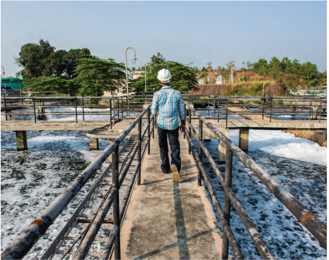
Karnataka Urban Development and Coastal Environment Project - Kavour Sewerage Treatment Plant.
