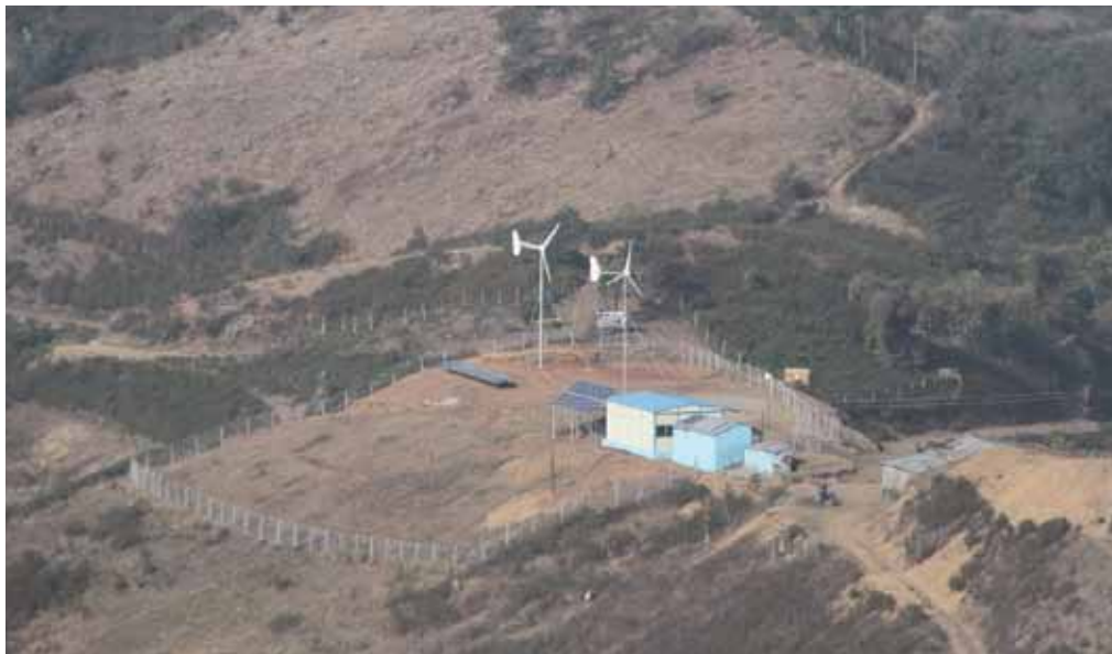
The two wind turbines installed at Dhaubadi, Nepal.
