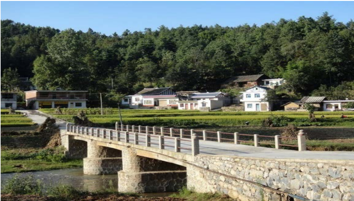
Roads in the village after the pilot project (photo by project team).
