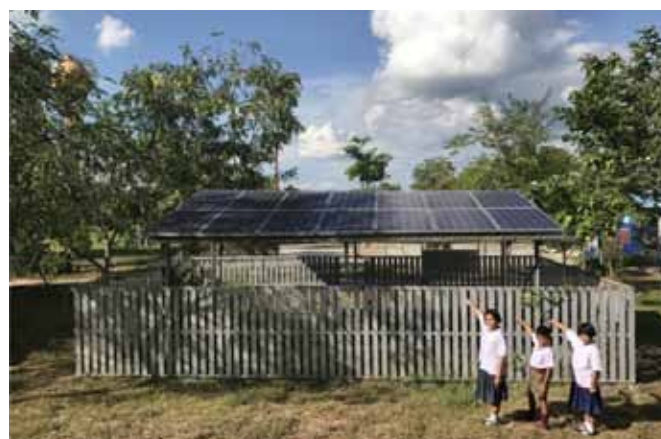
Solar panels donated by the NED to Bankhaotein school. Photo credit: National Energy Development.
