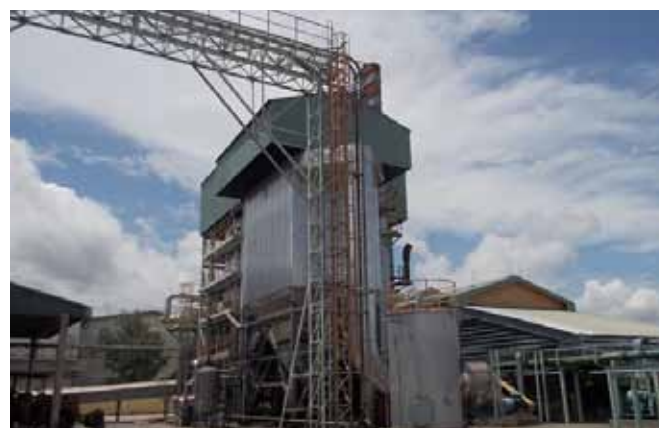
Angkor Rice Mill installed a 2-megawatt electricity generator which uses rice husk as a renewable fuel source. Photo credit: Future Carbon Fund.
