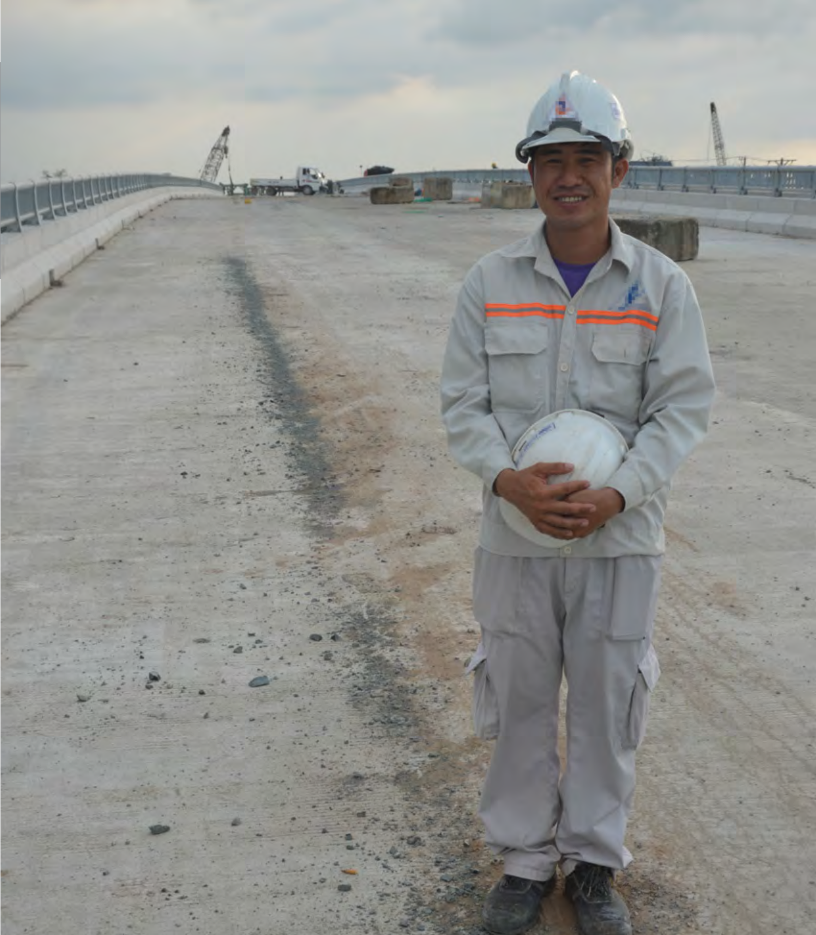
A site supervisor at the An Binh Interchange: The contractor's staff are often the first point of contact for complainants (photo by Nitish Jha).
