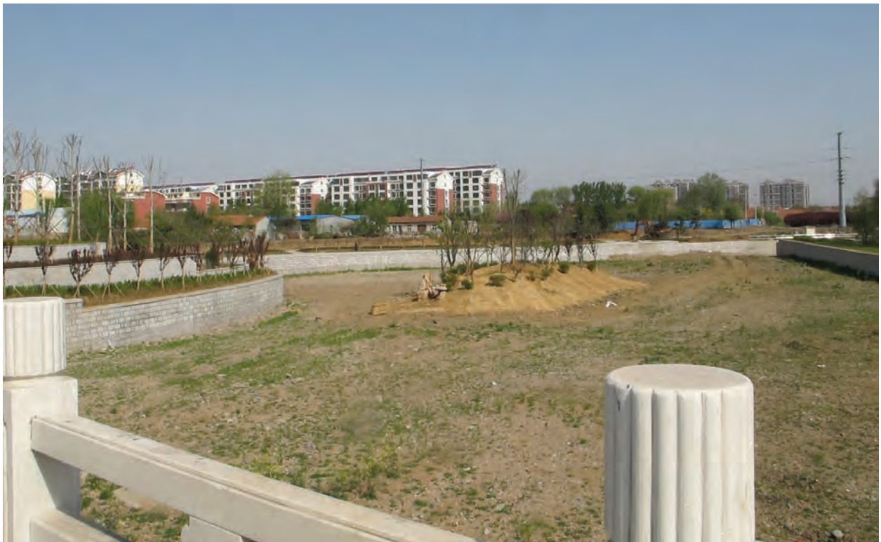
2. Branch of the Hucheng River at Yangzhou Road Bridge
