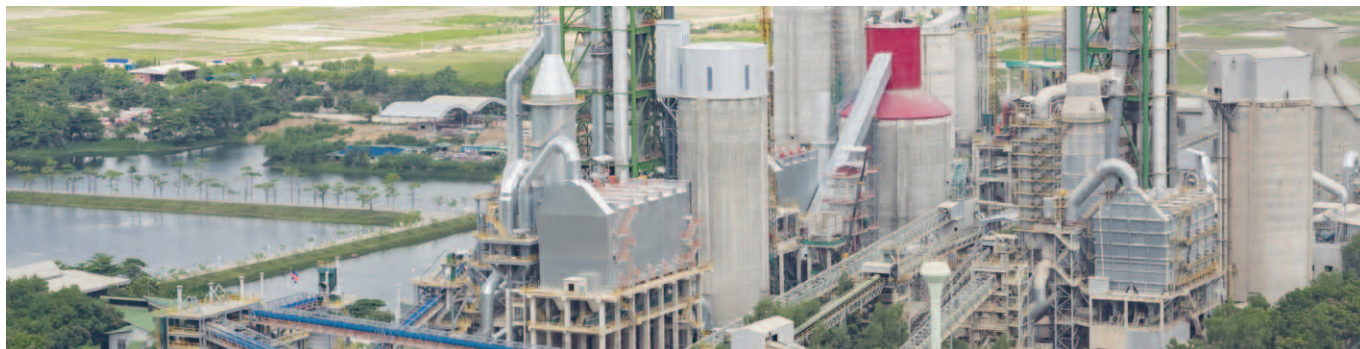
▲ A large cement factory under construction.
