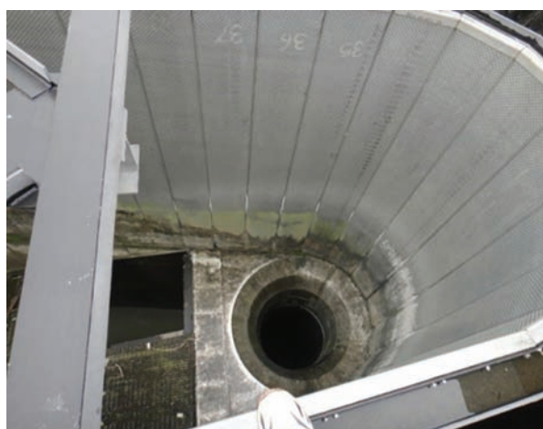
One-way fish outlet funnel in the dam of the Kali Gandaki A Hydropower Project. Fish are attracted toward the funnel by using fish-attracting light (photo by D.B. Singh).
