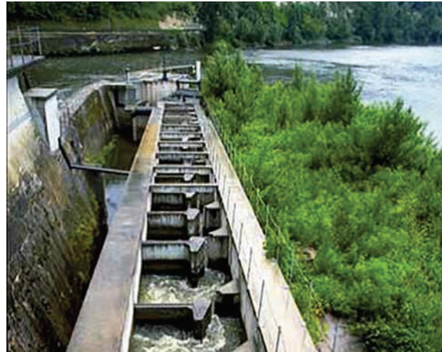
Typical example of fish ladder. If well-designed to different hydraulic criteria, a fish ladder provides passage for most fish species (photo by the Food and Agriculture Organization of the United Nations).
