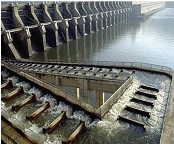
Pool-type fish ladder. The pool-type fish passage is an old concept, wherein the height to be crossed by the fish is divided into several small drops and forms a series of pools (photo by the United States Army Corps of Engineers).
