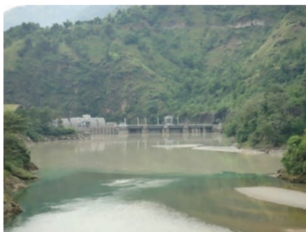
Dam of Kali Gandaki A Hydropower Project. A fish outlet funnel is provided for fish passage from upstream to downstream of the dam (photo by D.B. Singh).
