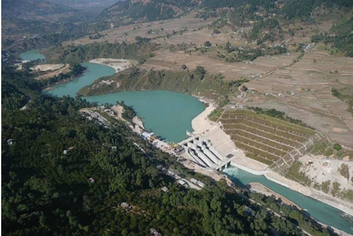
Middle Marshyangdi Hydroelectric Project (MMHEP) site. An aerial view of the MMHEP dam, which has no fish pass or fish ladder (photo by Bijaya.Ad).
