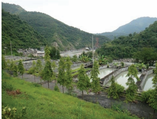
Fish hatchery of Kali Gandaki A Hydropower Project. Fish hatcheries try to compensate for fish stocks affected by dams (photo by D.B. Singh).
