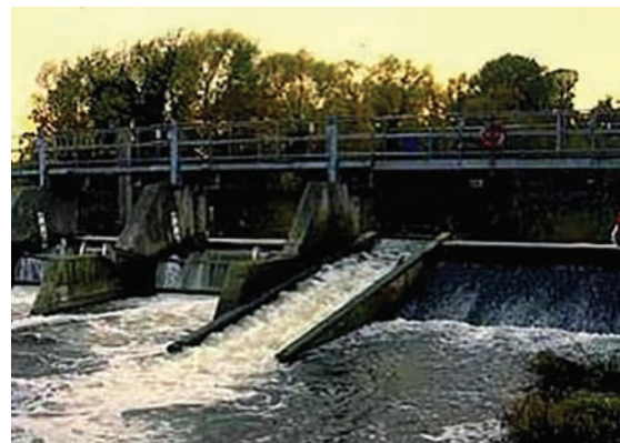
Denil fish passage. This type of pass is relatively selective depending on the fish species because it has no resting zone (photo by the Food and Agriculture Organization of the United Nations).
