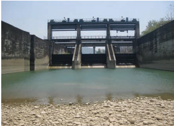
Irrigation dam of Babai. The Babai Irrigation System diverts water for irrigation through a barrage (photo by D.B. Swar).
