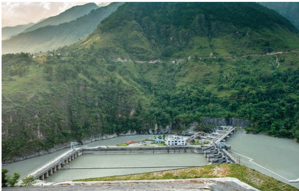
Kali Gandaki A Hydropower Project showing dam and desilting basin. The Kali Gandaki A Hydropower Project has a desanding reservoir at the downstream of the dam (photo by Samir J. Thapa).
