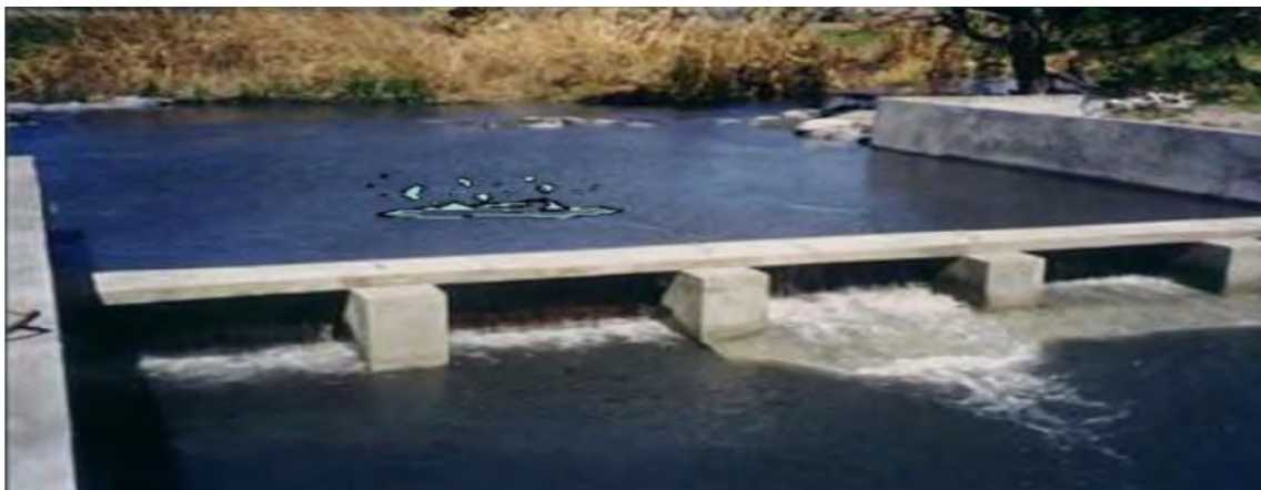
Small Diversion Dam (SDD)
