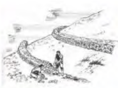
Erosion Control Bunds
