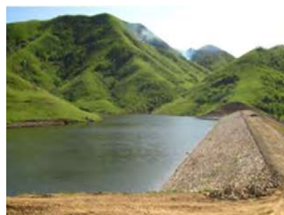
Shallow Well Impounding Project (SWIP)
