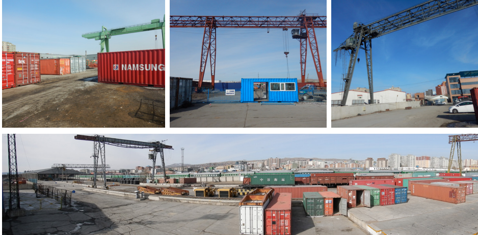
Various freight terminals in Ulaan baatar. Terminals have overhead gantry cranes, warehouses and are connected by a dedicated railway line.
