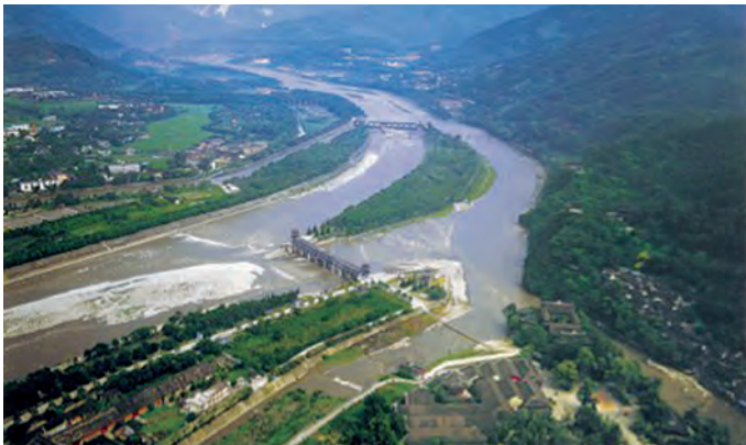
Dujiangyan (People's Republic of China). Waterworks facility supporting the development of Sichuan Basin from ancient times (photo by Sichuan Province Dujiangyan Management Office).
