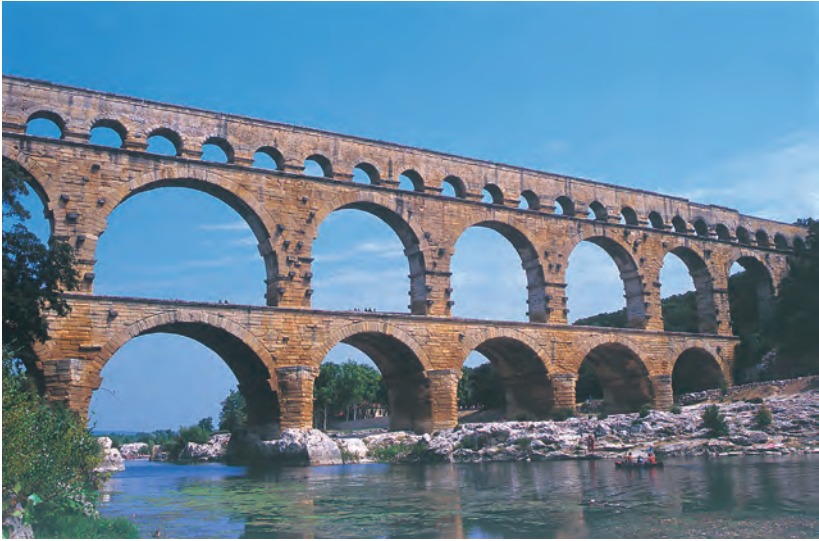
Pont du Gard (France). This ancient Roman aqueduct crosses the Gardon River in southern France (photo by Shigeo Hatsushiba).
