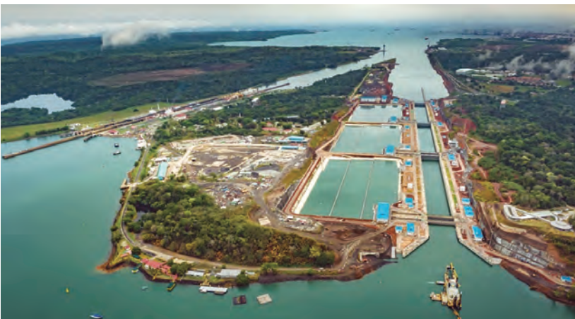
Panama Canal's Gatun Locks (Panama). The lock system allows ships to travel up and down the canal (photo by Panama Canal Authority).
