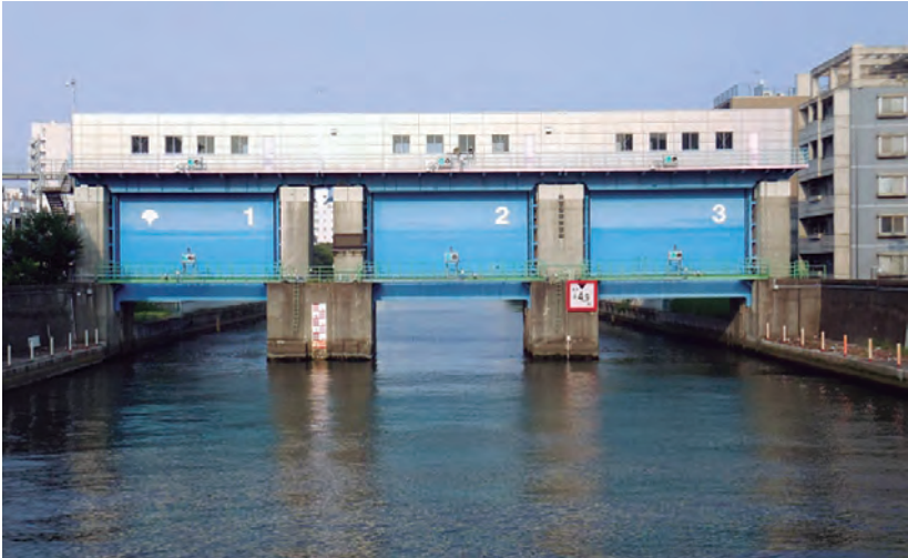
Shin-Onagi river water gate (Japan). These gates are meant to delay flooding and buy time for evacuation in the event of a tsunami (photo by Tokyo Metropolitan Government, Bureau of Construction).
