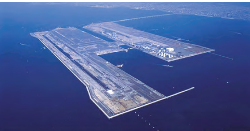
Kansai International Airport (Japan). The depth of the reclaimed land for this airport is particularly deep (photo by Ministry of Land, Infrastructure and Transport Civil Aviation Bureau).
