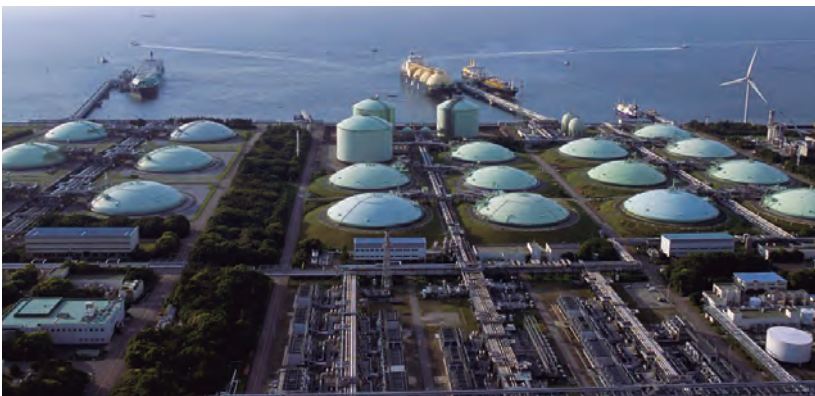
Sodegaura Liquefied Natural Gas Terminal. Liquefied natural gas is transported by sea at minus 162°C (photo by Tokyo Gas Co., Ltd.).
