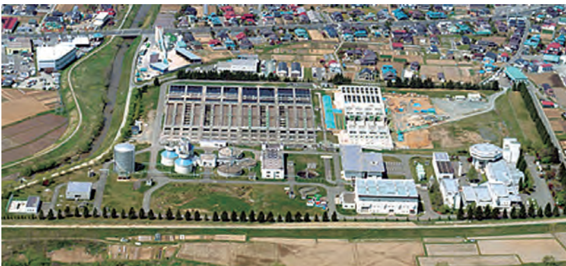
Tonan Purification Center (Japan). This center processes sewage in Morioka City (photo by Iwate Prefectural Sewerage Public Corporation).
