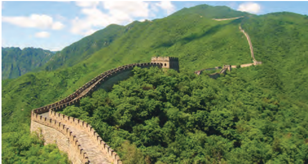
Great Wall (People's Republic of China). The wall was conceived as a defensive infrastructure to strengthen the territory and protect the country from invasion.
