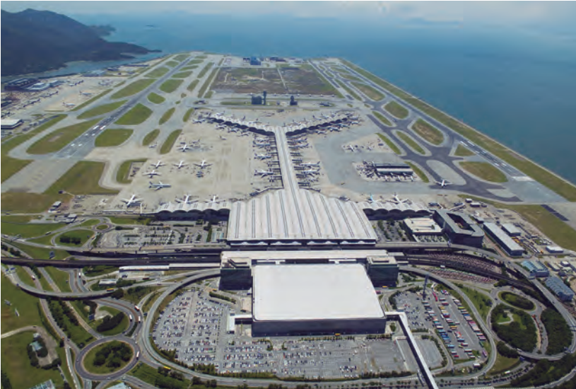
Chek Lap Kok International Airport (Hong Kong, China). Dozens of airports have been built on reclaimed land (photo by Hong Kong International Airport).
