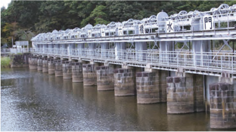
Asaka Canal/16 Bridge Gate. This was the first project publicly financed by the Meiji government (photo by Yūichi Nakamura).
