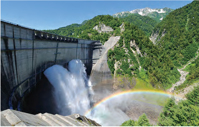
Kurobegawa No. 4 Hydro Power Plant. This project not only provided needed energy but also brought tourists to a previously hidden area.
