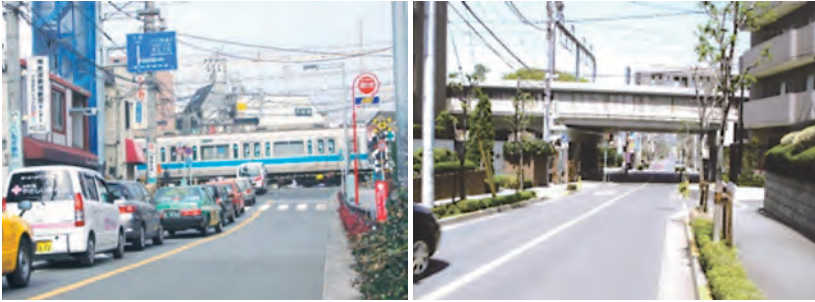
Multilevel Crossing Project (Kyōdō, Odakyū Line). Projects like these alleviate traffic congestion and make the urban landscape more cohesive (photo by Odakyū Electric Railway Co., Ltd).
