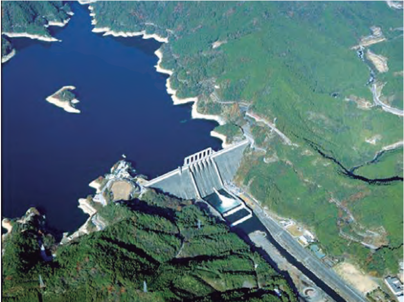
Sameura Dam (Japan). This dam is called the “water jar” of Shikoku (photo by Japan Water Agency, Ikeda Integrated Operation and Maintenance Office).
