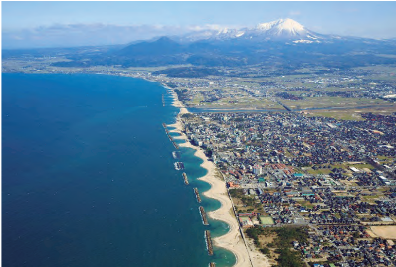
Kaike Coast (Japan). Various measures are used to combat coastal erosion, like these wave-dissipating blocks in Tottori Prefecture (photo by Ministry of Land, Infrastructure and Transport Hino River Office).
