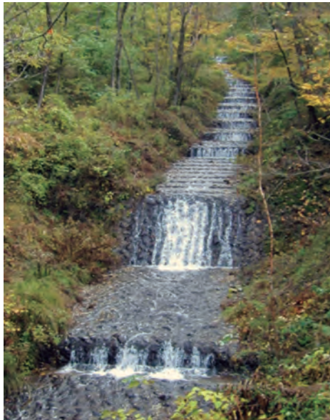
Stepped waterway of Ushibuse River (Japan). Stepped waterways like this one in Nagano Prefecture help to mitigate erosion (photo by Takeshi Yoneoka).
