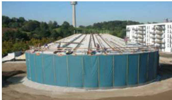
Figure 9: Underground Tank Thermal Energy Storage
