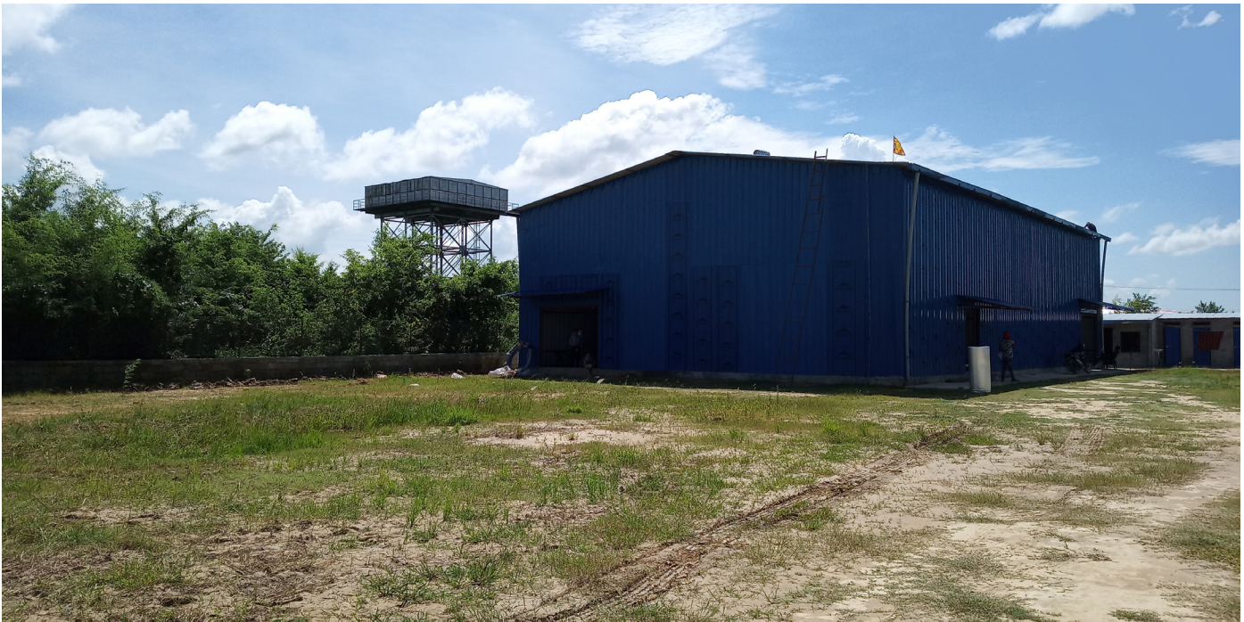
Construction site of one of the industries.
