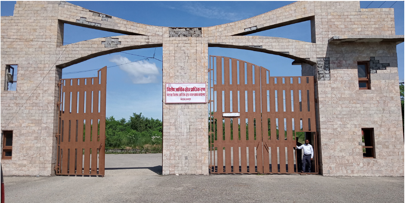
Main entrance to Special Economic Zone Authority, Bhairahawa.
