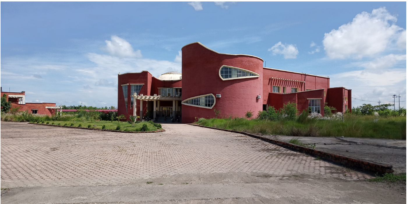
Main office building of Special Economic Zone Authority, Bhairahawa.
