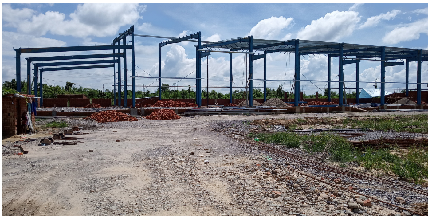
Construction site of one of the industries.
