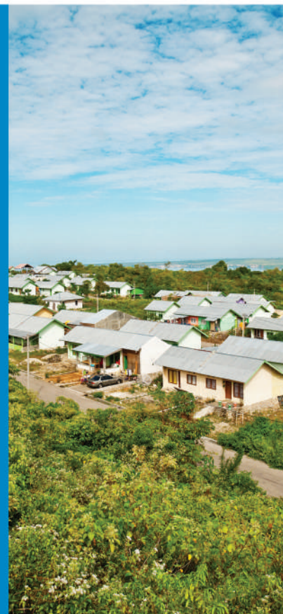
Low cost housing village built through the Neighborhood Upgrading and Shelter Sector Project in Bau-Bau, Buton, Indonesia (photo from ADB).
