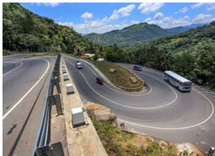
The Kandy–Mahiyangana national highway in central Sri Lanka was upgraded under the ADB-supported National Highways Sector Project.
